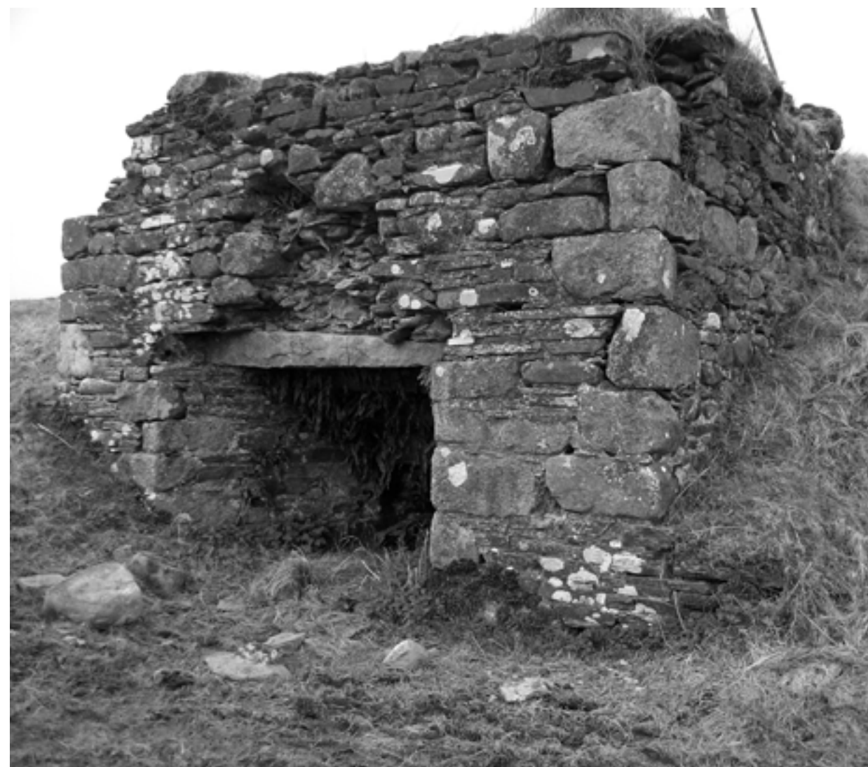
Figure 45: A typical lime kiln that made the limestone, built near the Canal used to build the royal canal itself and Mills such as Ashtown mill.
