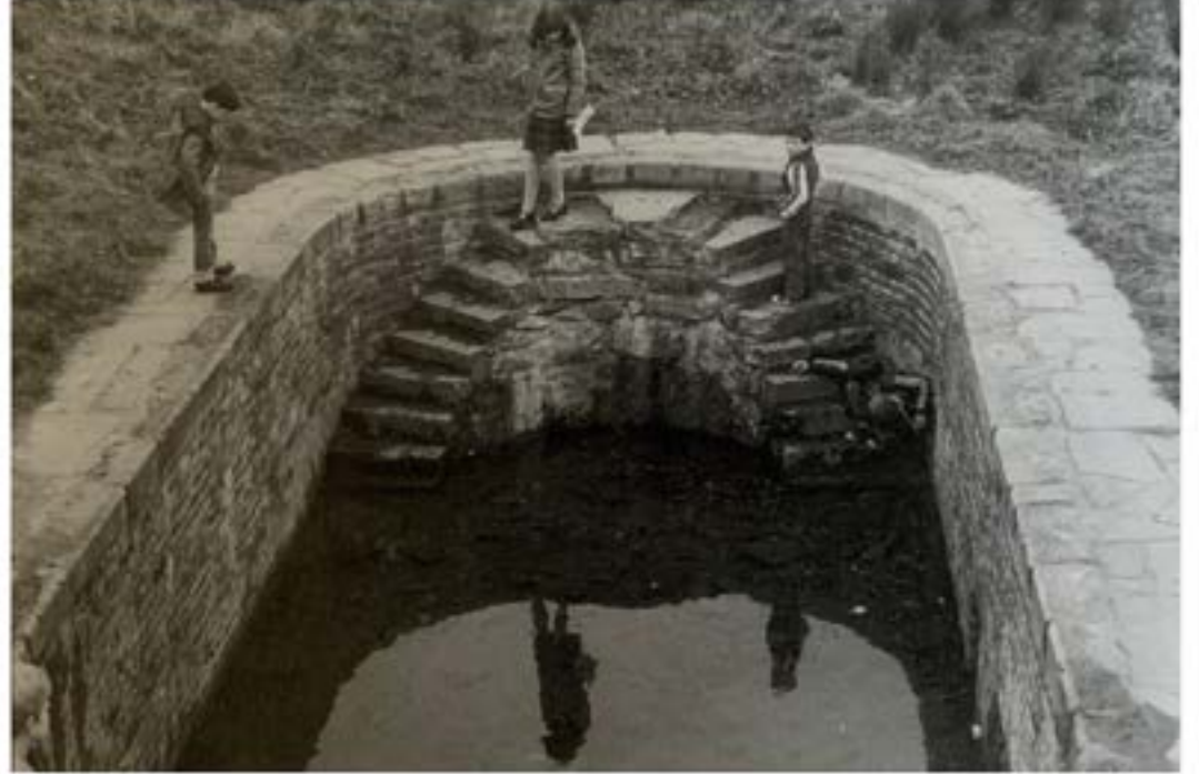
Built of finely cut limestone, were recreational features on the canal, such as the Romanesque bathing spa (c1794) in Leixlip next to the Rye Water Aqueduct, now disused. It was a popular health spa in the late 18th and early 19th century. Figure 42
