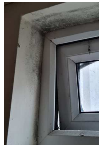
Mould in Kitchen Window Lintel
