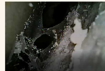
Inspection Camera inside the service cavity of Bedroom Wall
