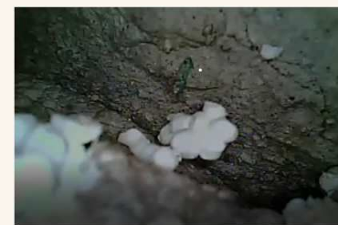
Inspection Camera inside the service cavity of Kitchen Wall
