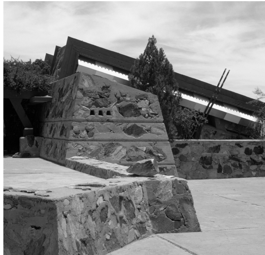
Fig 73; 'Desert Masonry', Taliesin West Building (Frank Lloyd Wright, 2019)
