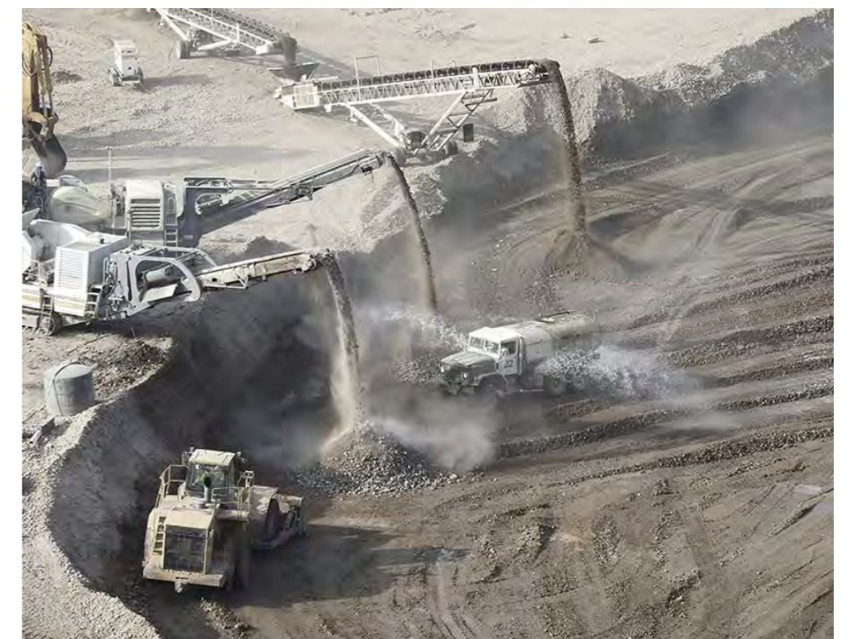
Fig 31; Backfilling Process (Geosolutions, 2020)
