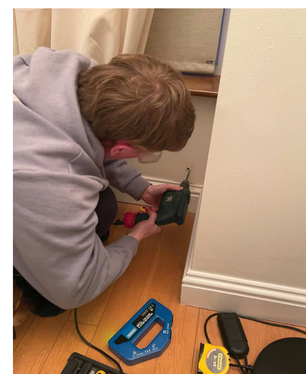
A hole was drilled using a 300mm drill bit. Care was taken not to drill into the external brickwork.
