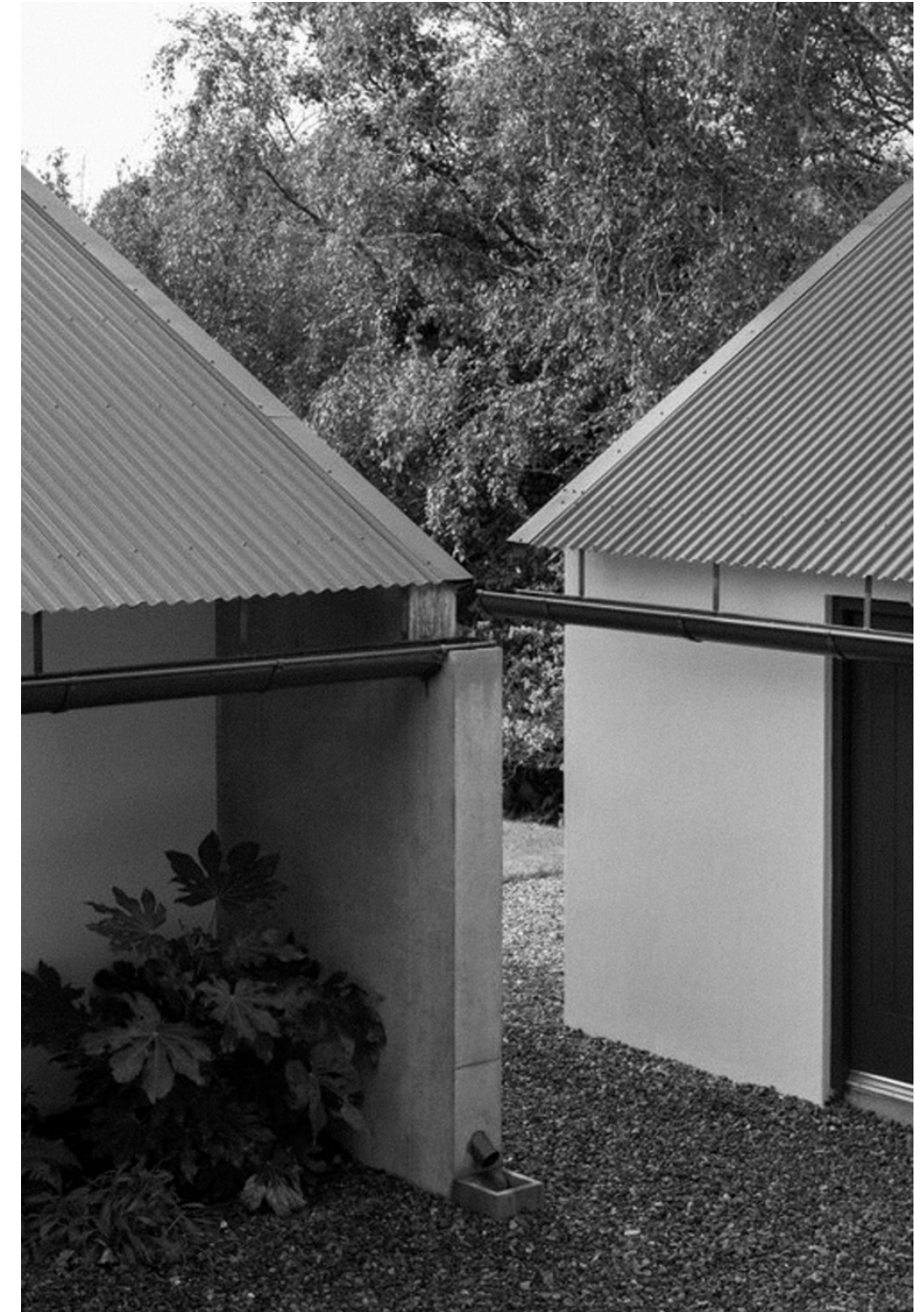
Fig. 15 Beach Road House, Gutter Detail
