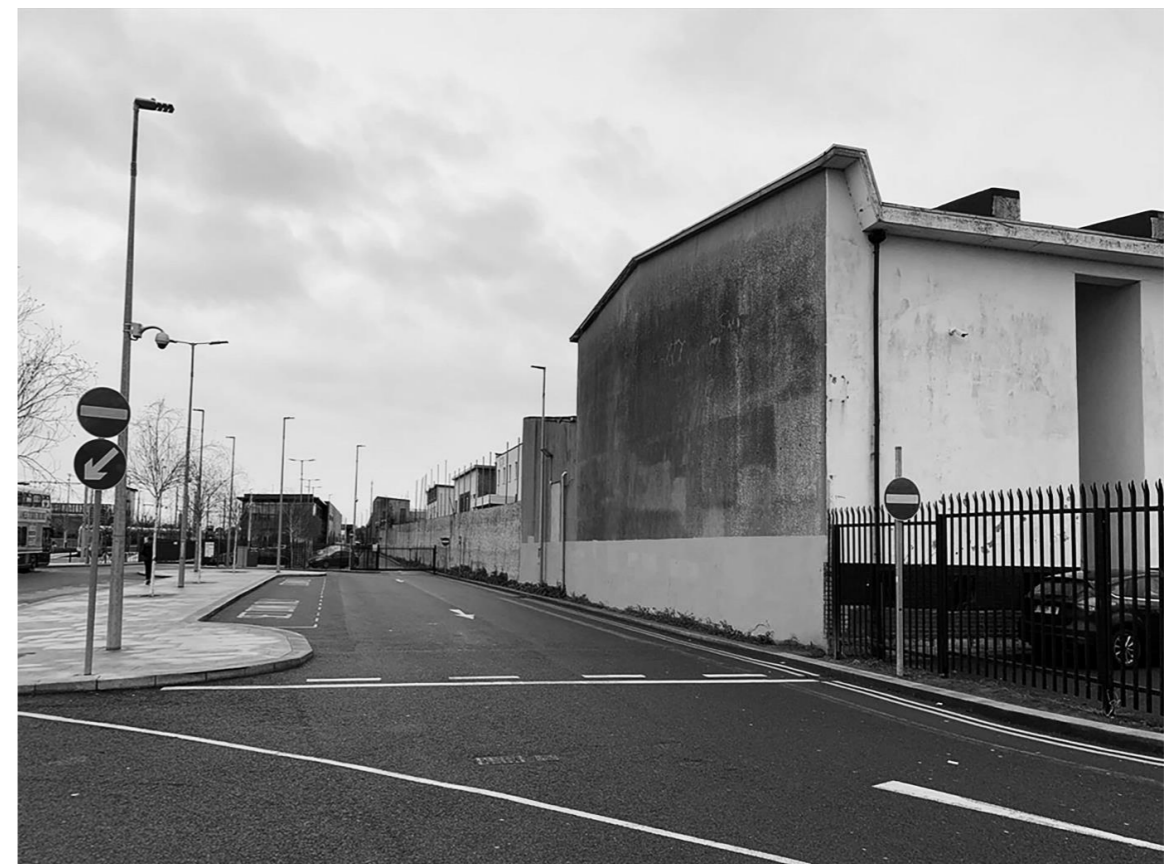
Photo of the building back
