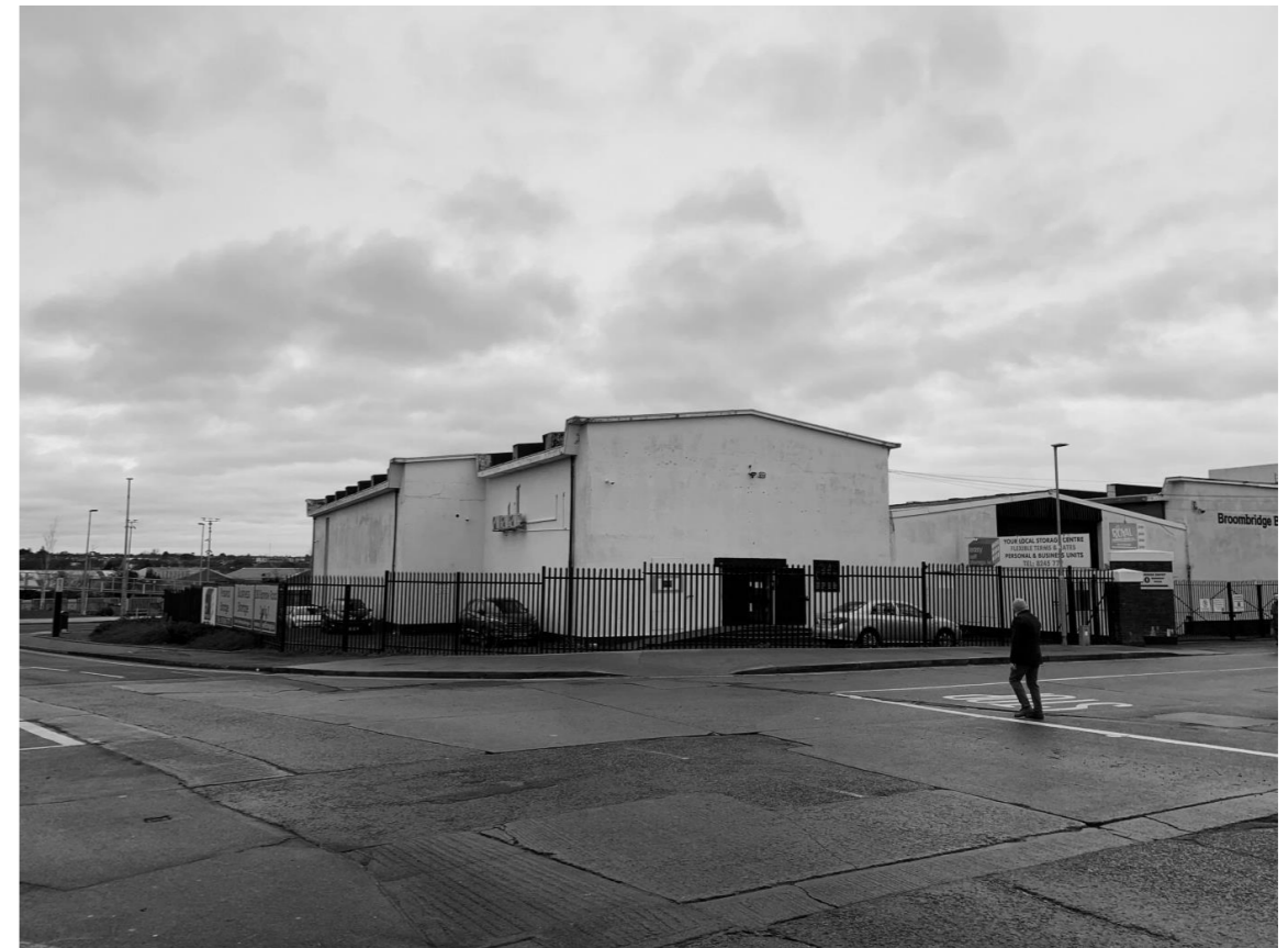
Photo of the building front
