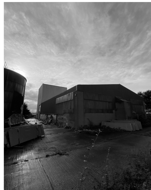
Fig. 9 & 10. Photographs - Building used to retrofit
