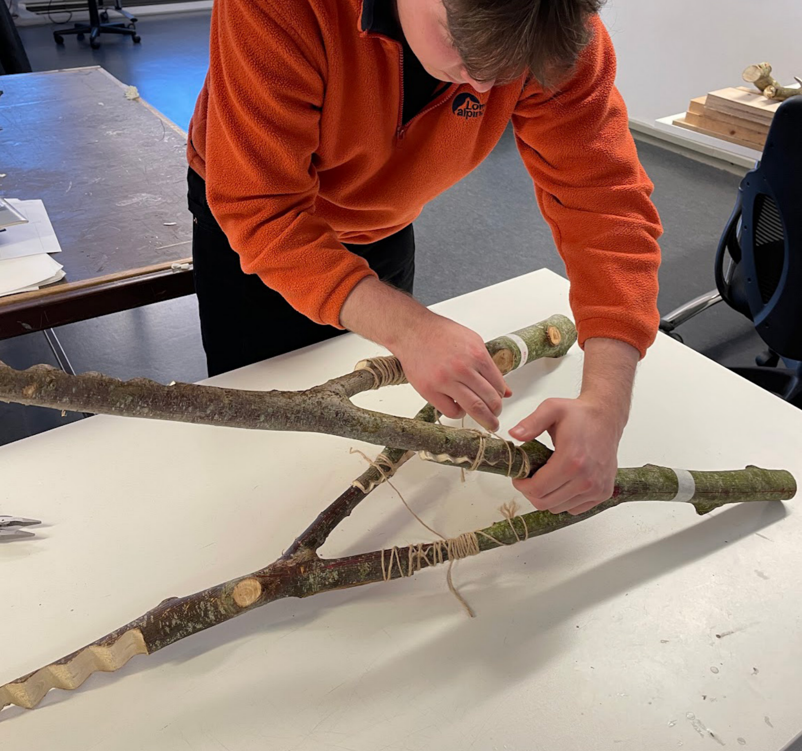
Figure 6.10: Assembly of the 4 branches to create the Tetrahedral Geometry | Nolan | 2015
