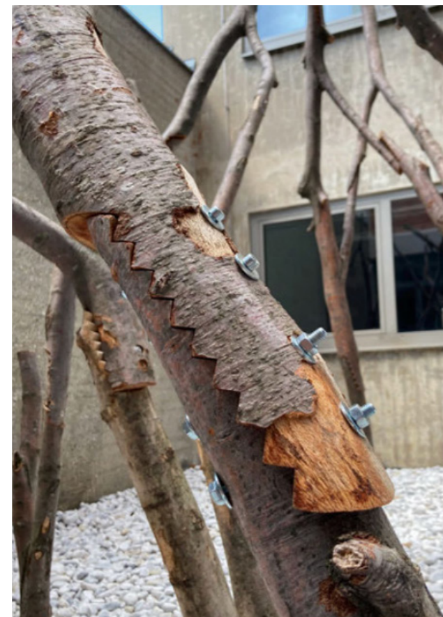
Figure 3.12: Nut and Bolted Connection | UAA Vienna | 2021
