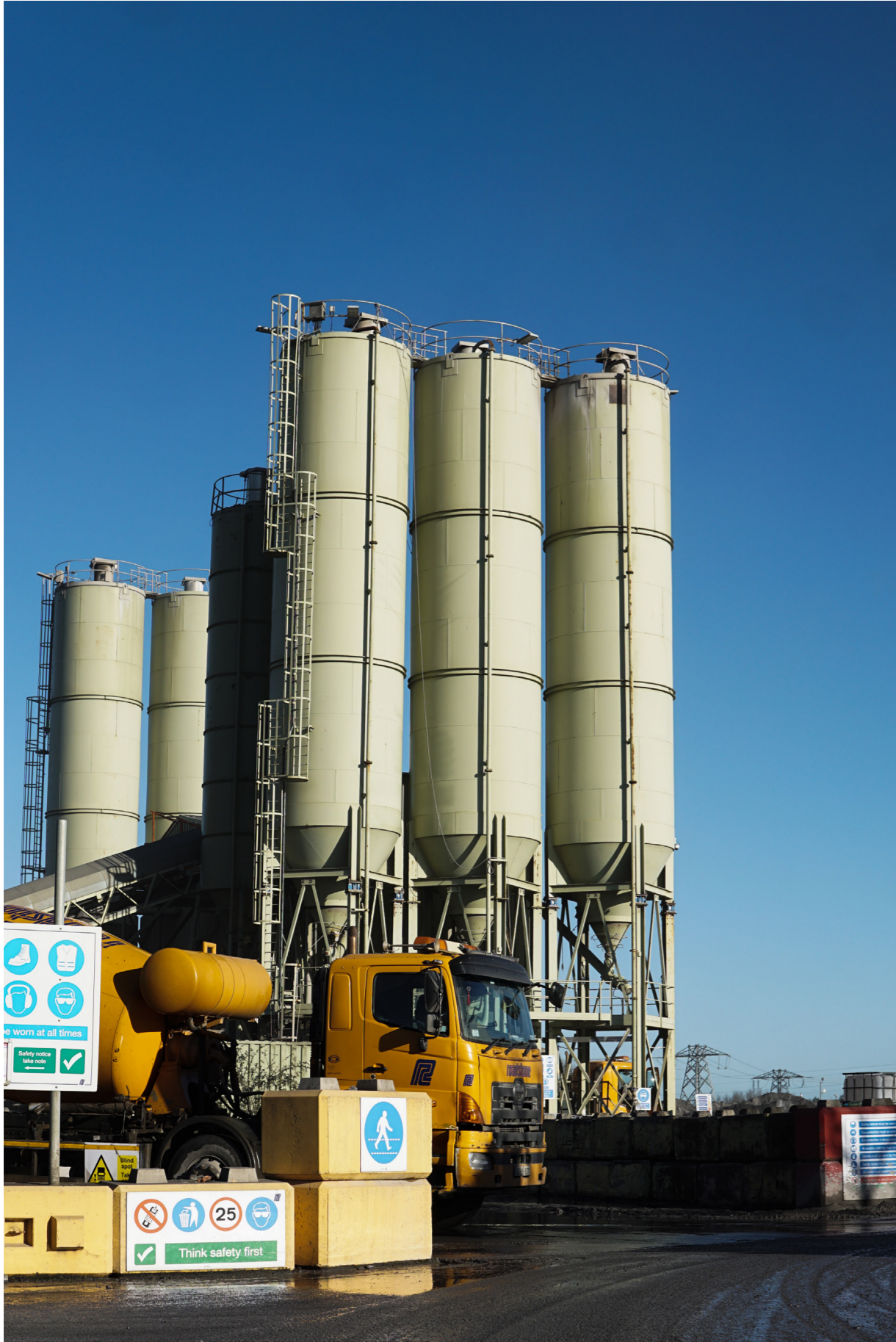
Figure 4.01: Huntstown Quarry Batch Mixing | Nolan | 2022
