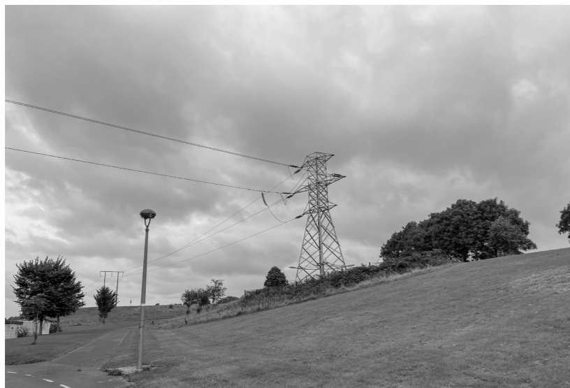
Above: Electrical Infrastructure in the park
