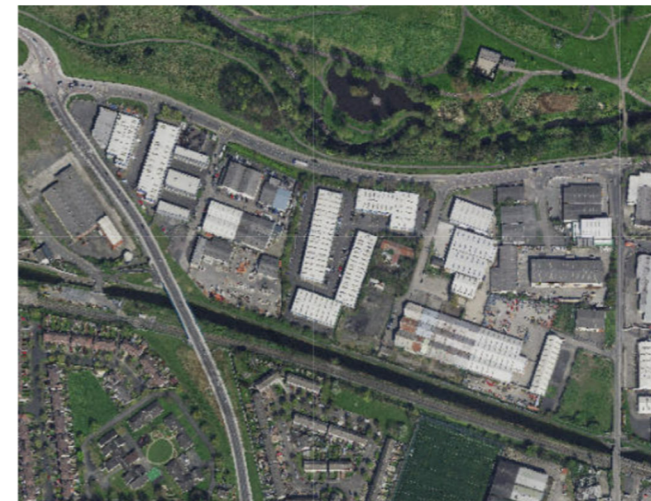
Fig.29. Site aerial 2013. Factory removed from site.
