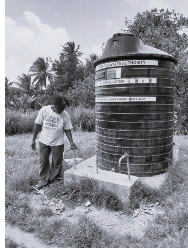
[fig 1] Mother and son at traditional standpipe bath (left) [fig 2] Man at community water storage tank (right) [fig 3], Visit to Seapoint beach, Dublin [fig 4, fig 5] Adjacent Blackrock Public Bath, in use, and now derelict respectively
