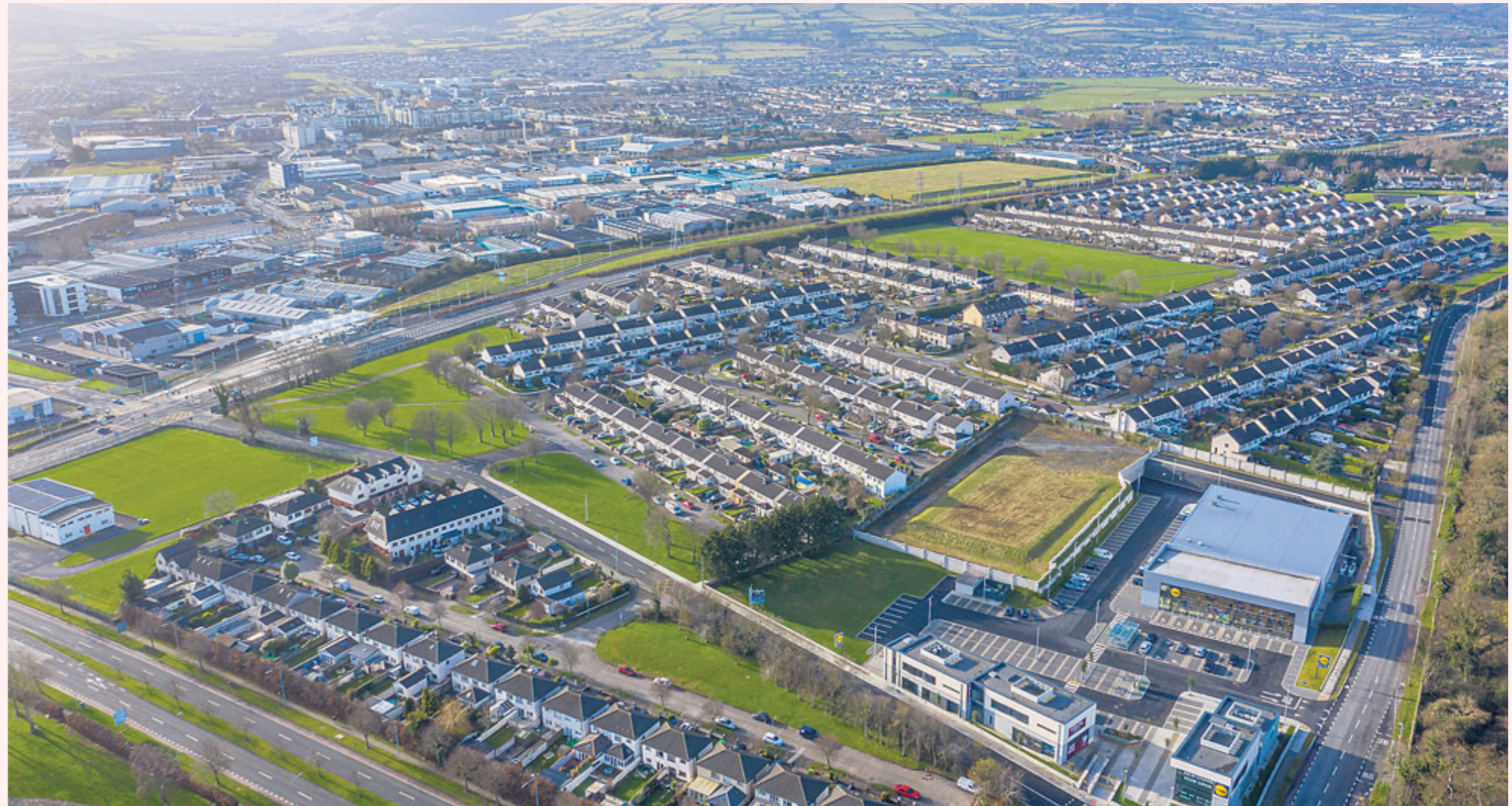
Fig. 13- Tallaght, one of Dublin's most dangerous places
