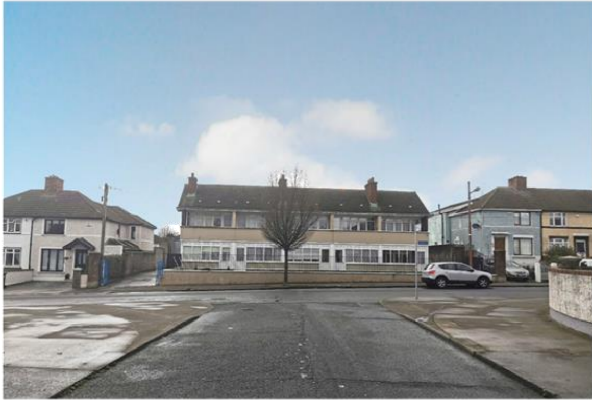
Existing Apartment Block
