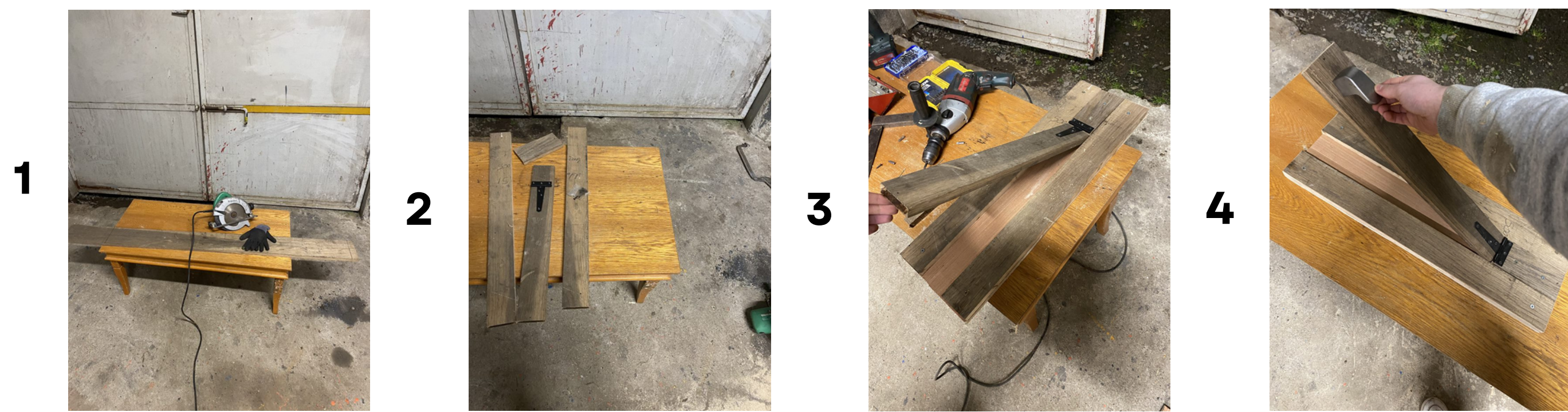
1 Wooden Floorboards were salvaged and a saw was sourced.
