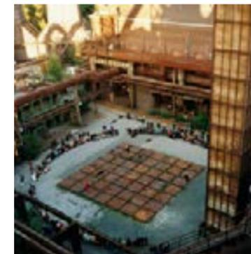
*cast iron plates reused as pavement
