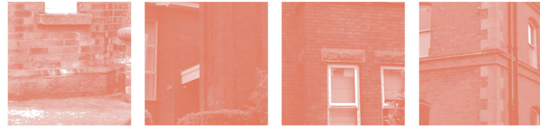
Some derelict stone/ashton brick buildings in cabra.
