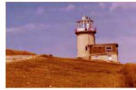
Fig.2.2 Belle Tout Lighthouse - Set Back 100 Feet - To Provide Clear Light
